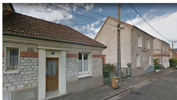
Fig.129 - Rue Louis Loucheur, Orléans Source : Google Street View
